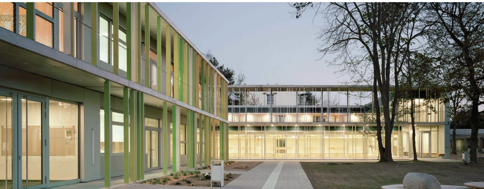
Project: Elementary school Karlsruhe, Germany; Architecture: Wulf Architekten; Photo: Brigida González
