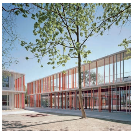
Project: Elementary school Karlsruhe, Germany Architecture: Wulf Architekten; Photo: Brigida González
