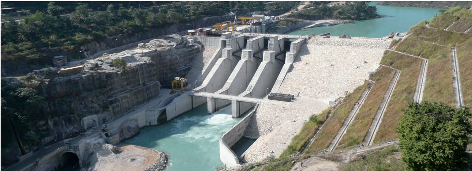
Project: Hydroelectric Power Plant Middle Marsyangdi, Nepal, Constructor DYWIDAG International GmbH
